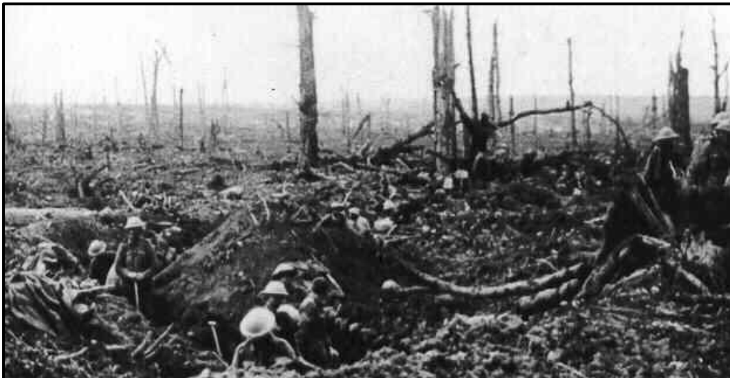
Trenches in Delville Wood in France during WW1
