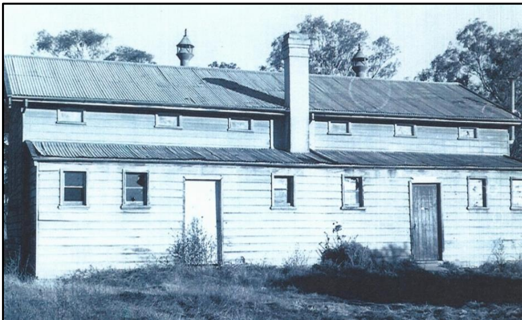
The original Hoxton Park Public School (Photograph courtesy of Liverpool City Library)
