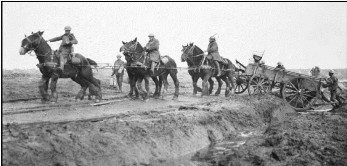
Six horses haul a General Service (GS) wagon from a ditch through slippery mud on a corduroy track in the Ypres sector in Belgium. (Australian War Memorial E01054)
